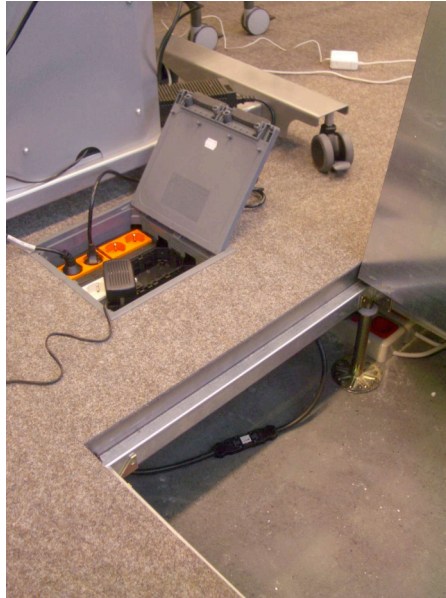
Fig. 7: An open floor panel in the Aachen Media Space. The entire panel including the floorbox can be moved.
